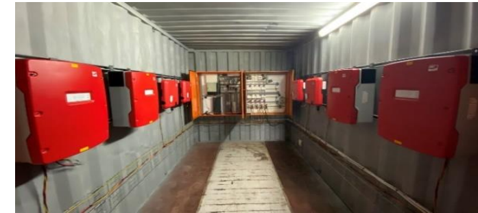
Containerised microgrid
