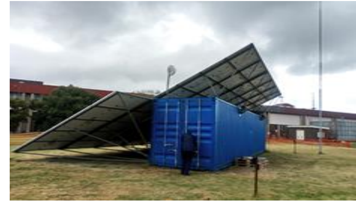
Containerised microgrid
